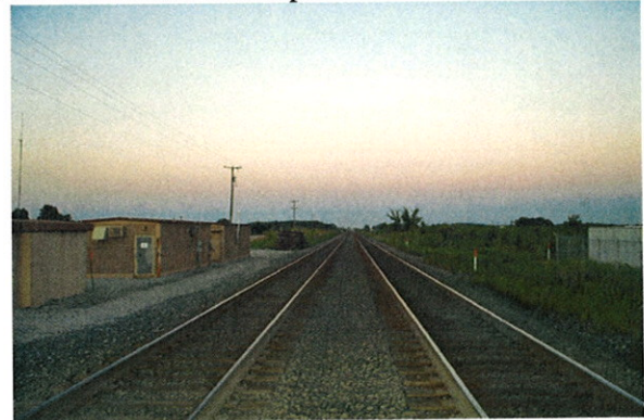
PHOTO 4: MP 364 at CR 47 looking east
