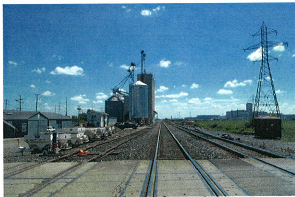
PHOTO 1: Looking east at Walnut Road crossing in New Carlisle, MP448.3 a proposed flyover location
