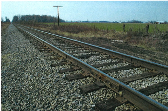
Photo 10: At County Line Road looking south
