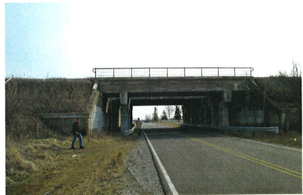
Photo 11: Looking east along the Indiana & Ohio Railway at County Road F
