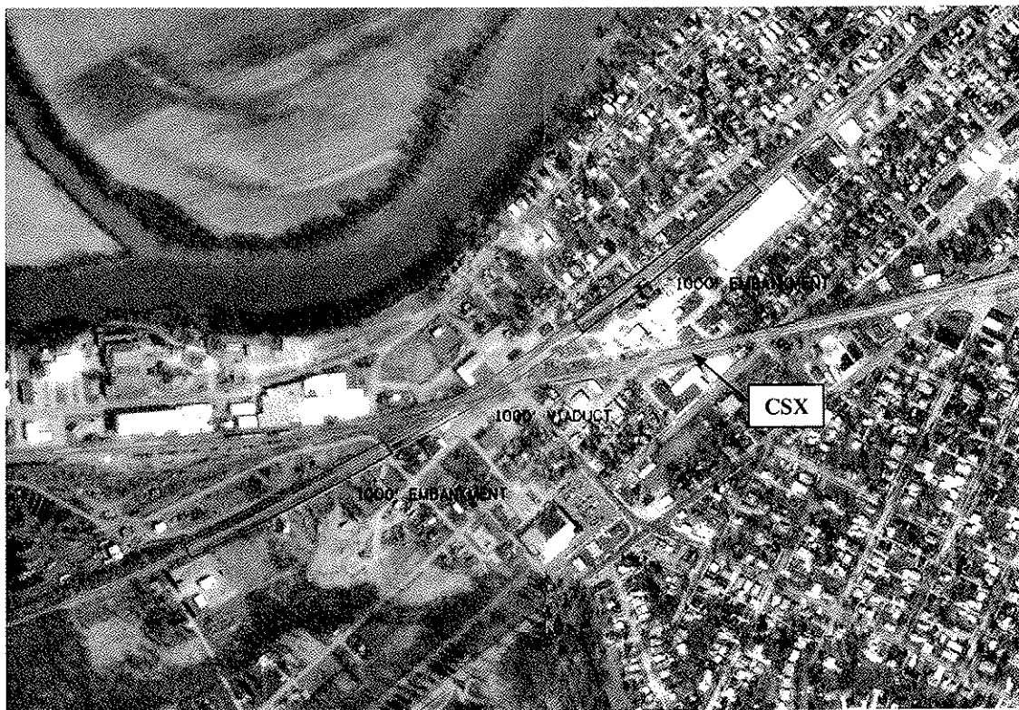
Exhibit 2-7: In Defiance, viaduct and embankment over CSX
