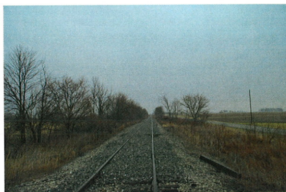
Photo 8: At Guston Rd. crossing near MP 77 east of Woodburn, looking east
