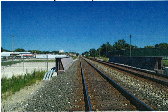
PHOTO 3: At MP 434.4 in South Bend, looking east
